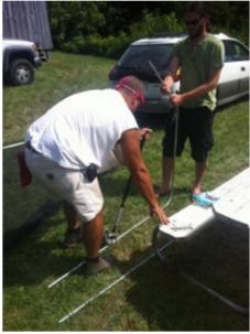
Here's one of our gardeners, Randy, learning how to bend a section of EMT conduit into a "rib" for his midtunnel frame.
